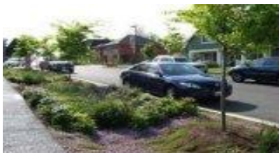
Bioswales are essentially rain gardens placed in long narrow spaces such as the space between the sidewalk and the curb.
