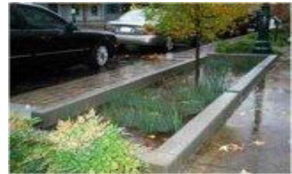
Planter boxes are an attractive tool for filtering stormwater as well as reducing the runoff that goes into a sewer system.
