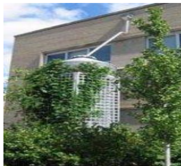
This rainwater harvesting system is adapted to the architecture of the building and its surroundings.
