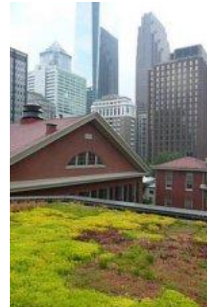
A green roof system atop a building helps manage stormwater and reduce energy costs for cooling.
