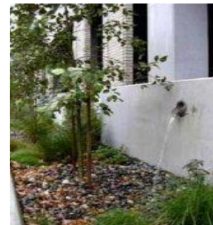
Water from the roof flows from this disconnected downspout into the ground through a filter of pebbles.
